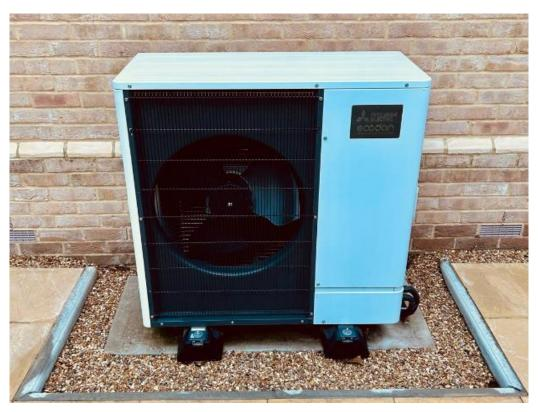
The condensate that accumulates can be guided into a sewer, pump sump or soakaway via a downpipe, gully, balcony run-off or roof run-off. Open gullies or downpipes within the protective zone do not pose any safety risk. For all installation types, you must ensure that any condensate that accumulates is discharged frost-free.
